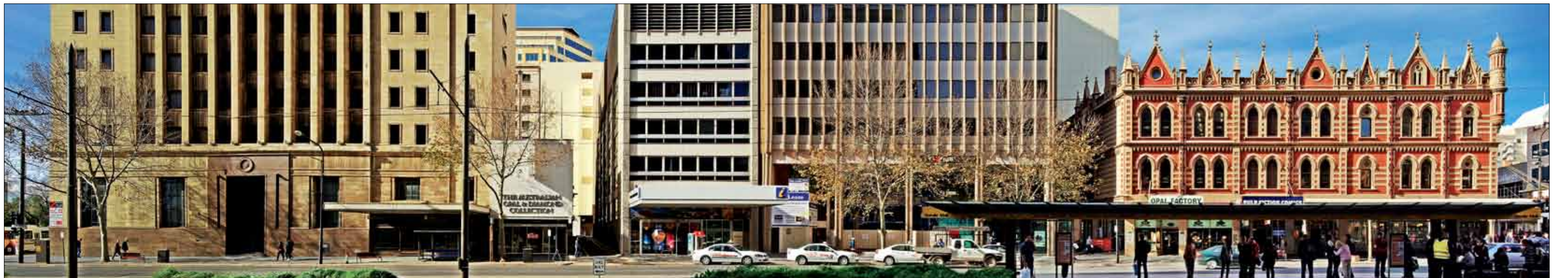
FORMER BANK OF NEW SOUTH WALES (1939-1942)
