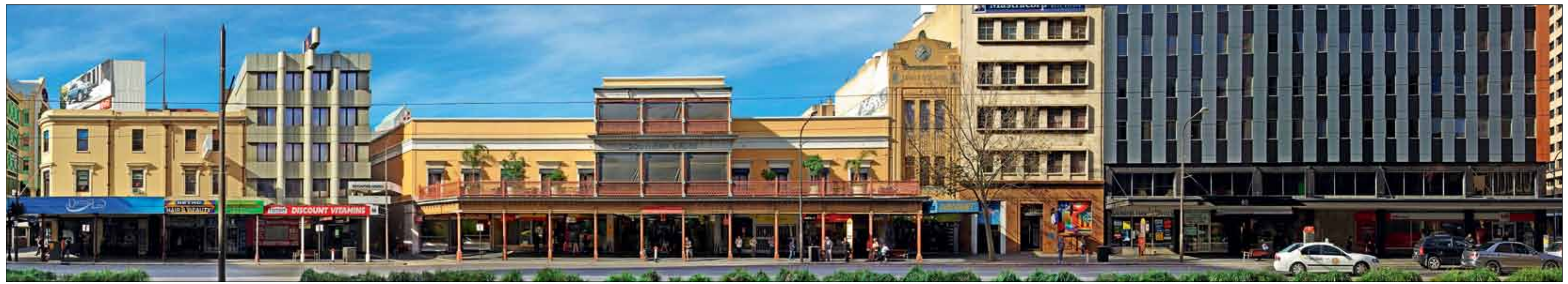
FORMER WATERHOUSE CHAMBERS (1848)
